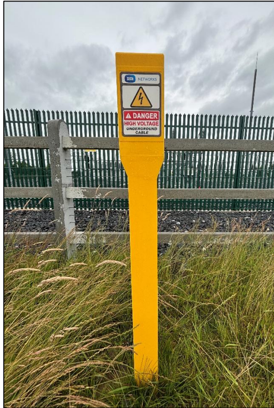
Figure 5-7 Typical Cable Marker Post
